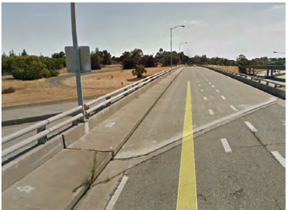
North Sand Hill Road overcrossing and sidewalk
