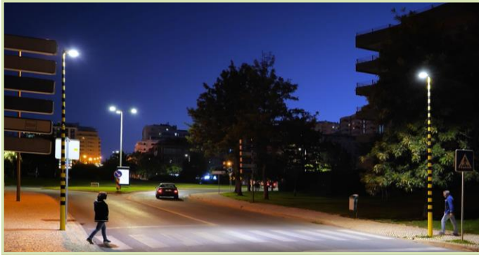
Sidewalk and crosswalk lighting
