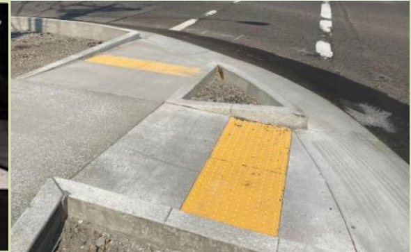
Accessible curb ramps
