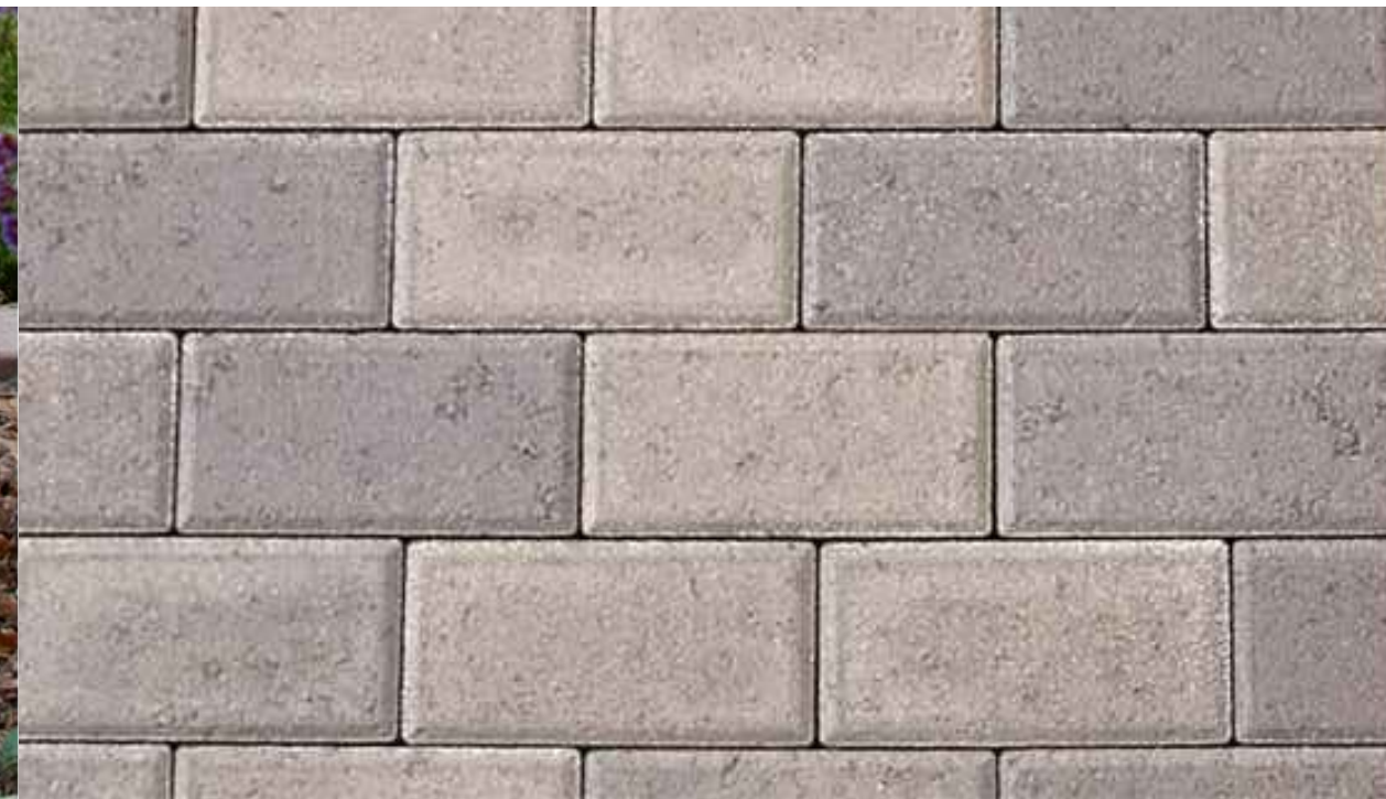
PERMEABLE PAVERS AT DRIVEWAYS (RUNNING BOND)
