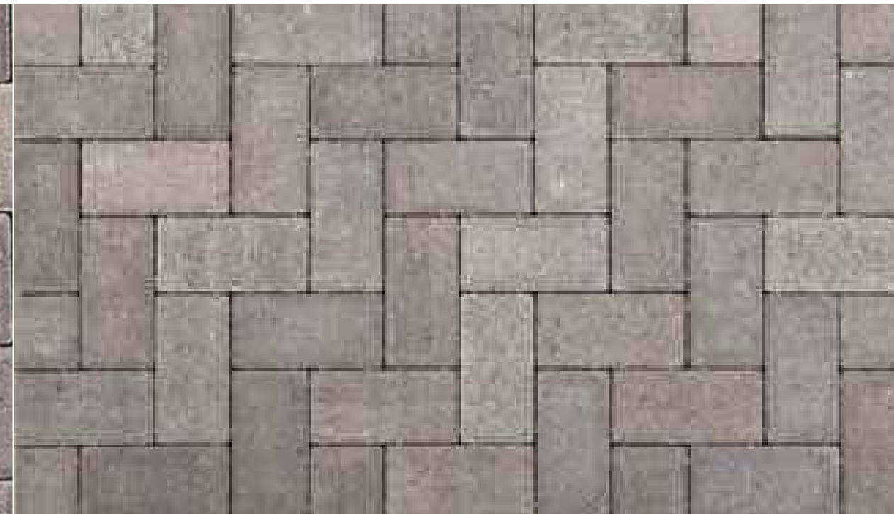
PERMEABLE PAVERS AT DRIVEWAYS (HERRINGBONE PATTERN)
