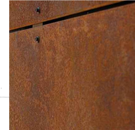
CORTEN STEEL PLATE AT ENTRY GATE AND GABION BENCH
