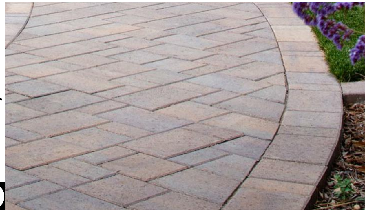
PERMEABLE PAVERS AT DRIVEWAYS (ASHLAR PATTERN)
