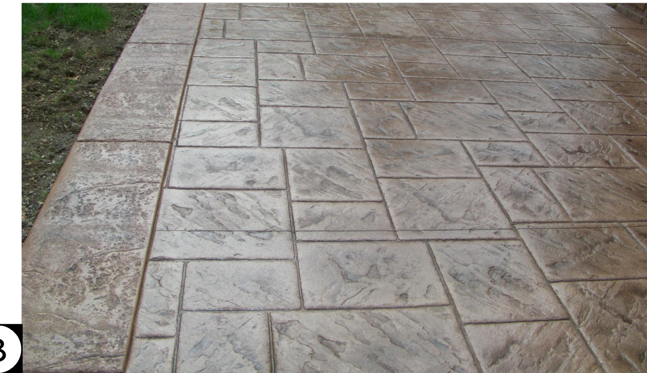
STAMPED CONCRETE AT DRIVEWAY ENTRANCES
