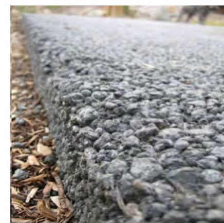
Pervious concrete step
